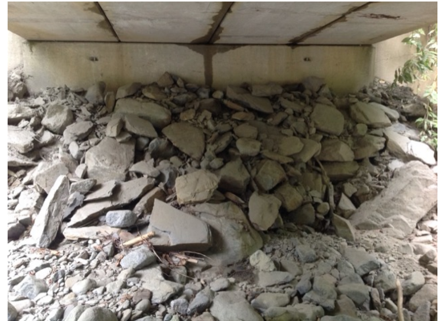
Left Bank Abutment when facing downstream
