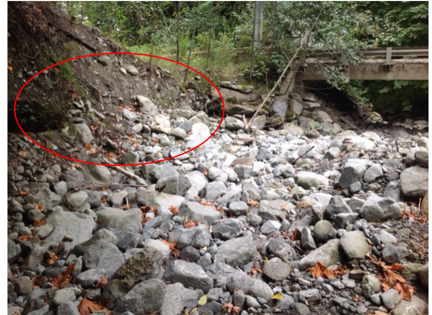
current hi flows are being directed towards left bank - behind riprap
