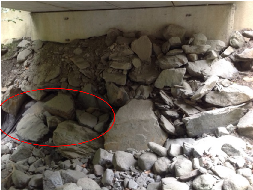
Right Bank Abutment when facing downstream
