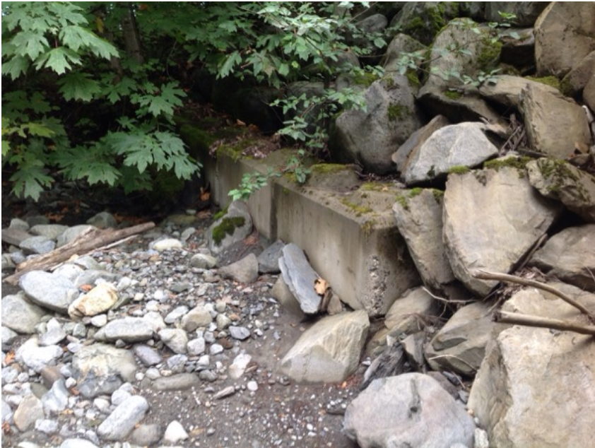
downstream right bank wing wall
