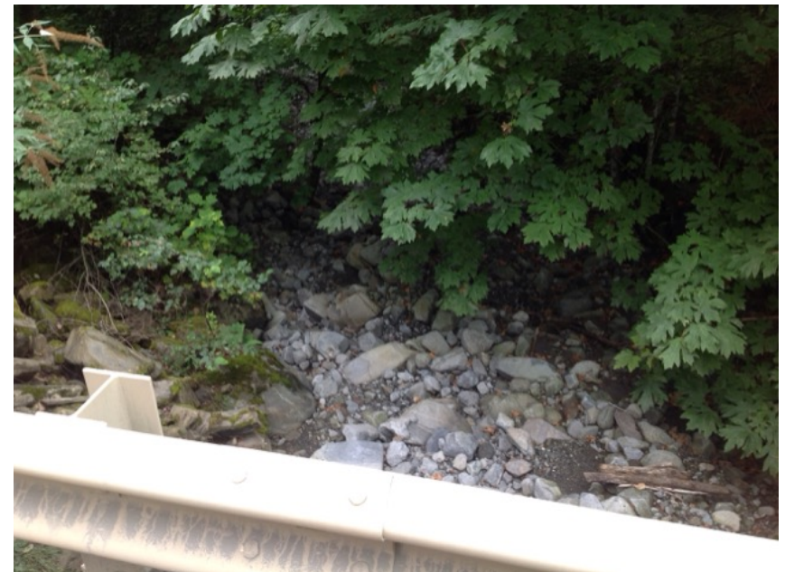
looking downstream from deck
